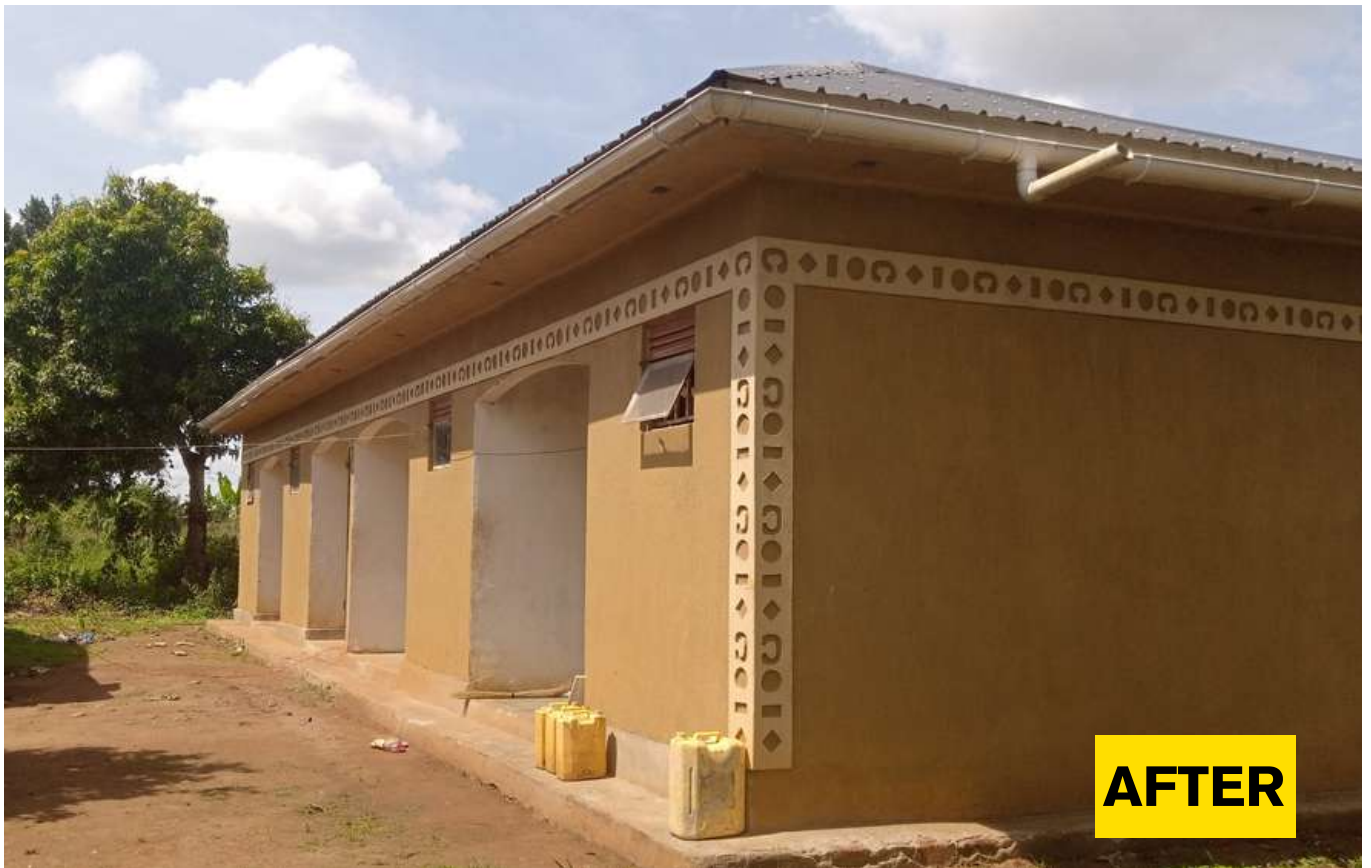
A teachers' quarter constructed at St Jude Muwangi Primary School in Luwero District
